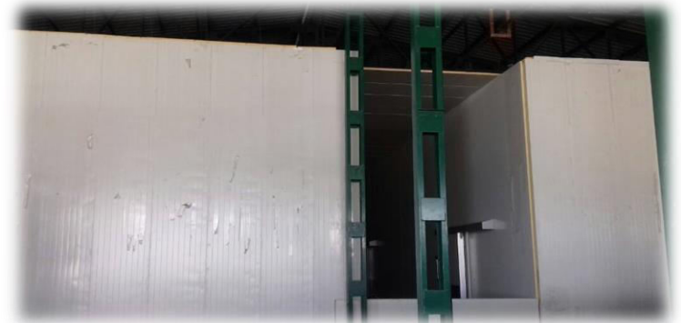
Storage chambers of -20 degrees with 2000 MT capacity
